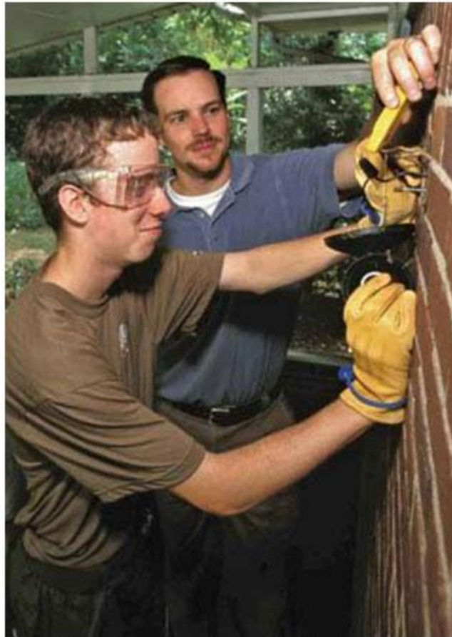
A Scout repairs a home electrical system
